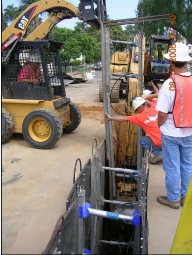
Fig. 6. Sequential shoring operations in fast-raveling sands.
