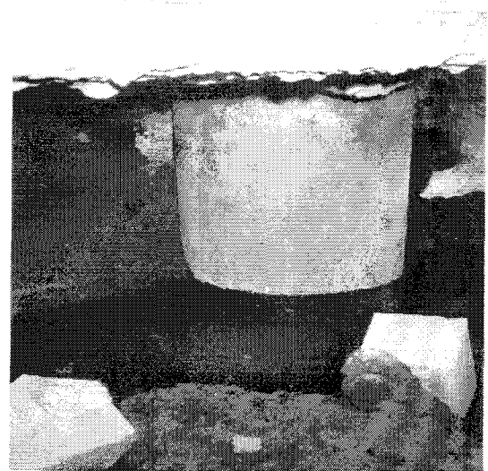
Fig. 7. Undamaged pile under ferry building in Port Island after Kobe earthquake, 1995.
