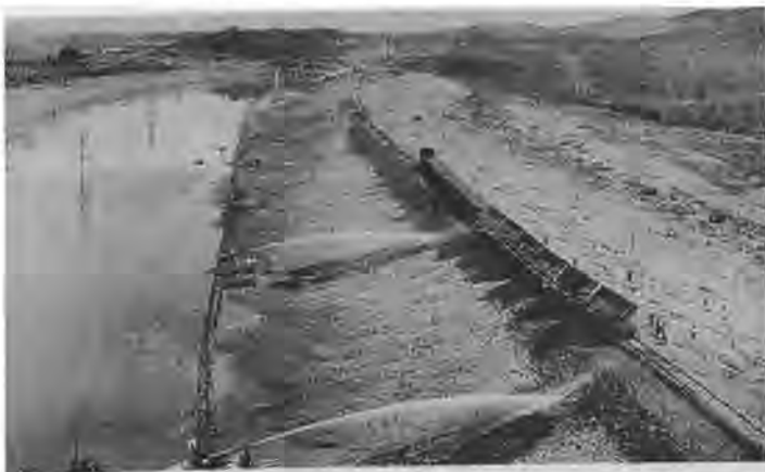
Photo 1 Embankment Construction: Material dumping and Water Jet Washing
