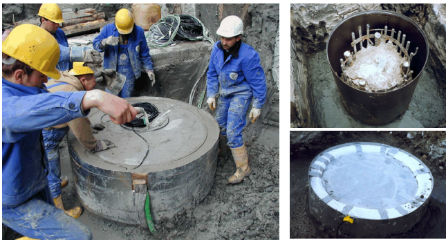
Fig. 15. Installation of a load cell on a pile head
