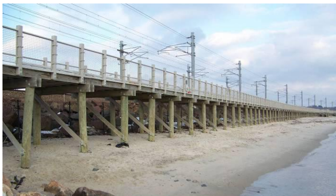
Photo 2. Original Boardwalk (looking east towards bridge)
