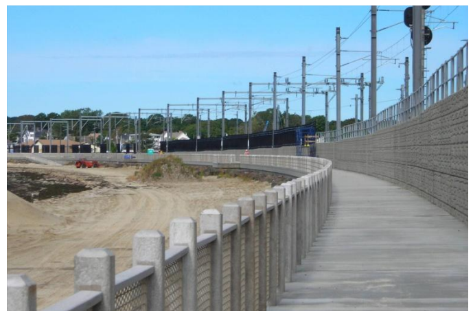
Photo 10. Completed Two-Tier Wall and Elevated Walkway
