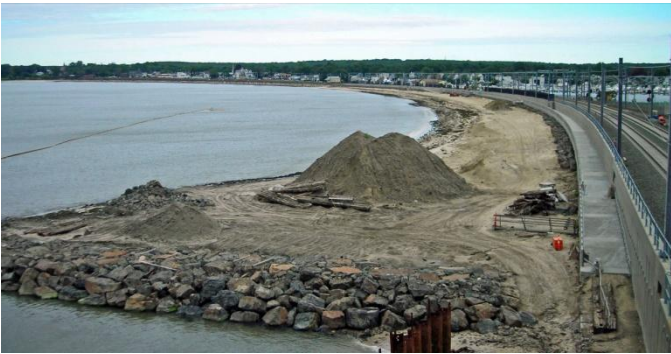
Photo 12. West Approach Wall, Ramp and Terminal Groin
