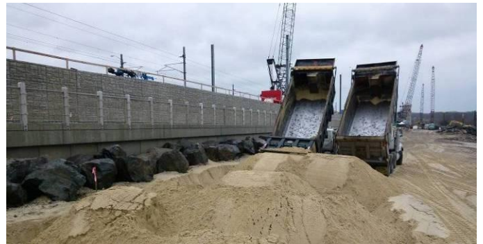
Photo 5. Placement of Sand for Beach Replenishment
