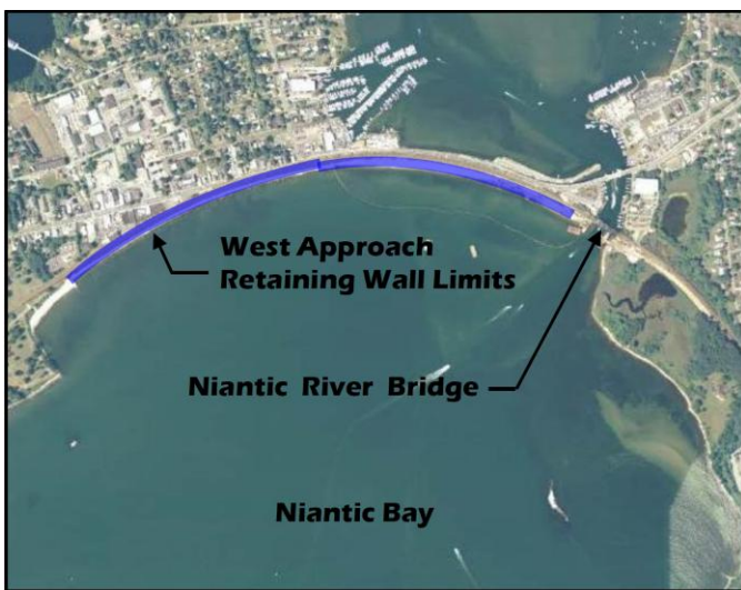
Fig. 1B. Site Aerial View with West Approach Wall Limits
