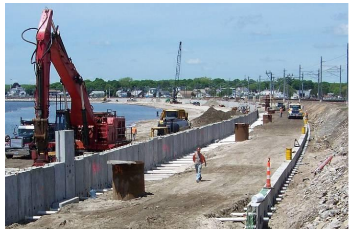
Photo 7. Continuous Deadman Construction
