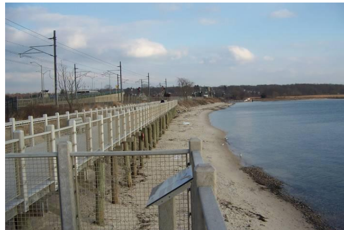
Photo 3. Original Boardwalk (looking east towards bridge)
