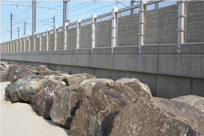
Photo 11. Wall with Close-up of Revetment Stones
