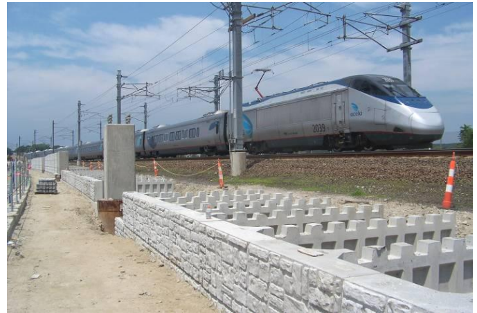
Photo 6. Wall Construction with Catenary Pole Foundation
