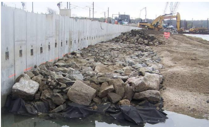
Photo 4. Installation of Scour Protection System
