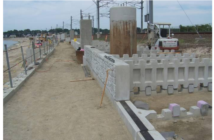
Photo 9. T-WALL Construction and Walkway Subgrade
