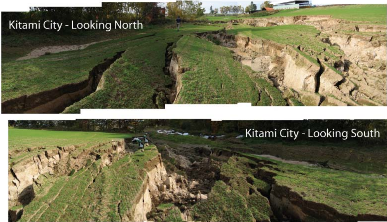
Figure 40: Flow failure in a farm field near Kitami City, where 5,000 to 10,000 m 3 of volcanic ash fill soil was expelled from a single site as a result of liquefaction (Photo Mosaic: R. Kayen).
