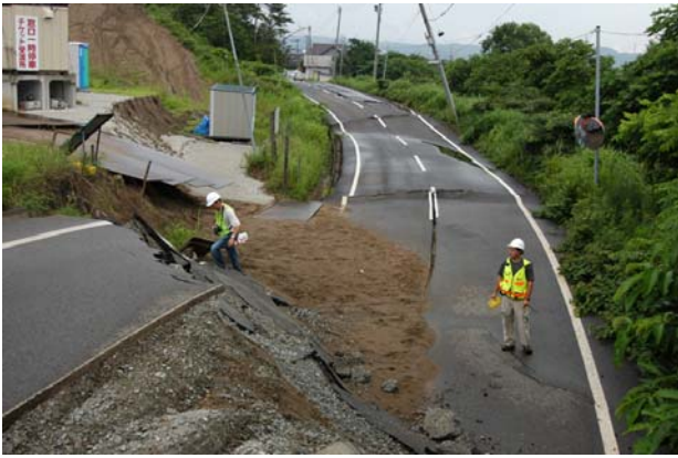
Figure 7: Lateral Spread on North side of Kai-Un Bridge area of the Sabaishi River (Google Earth map site RK6, N 37.39343 E 138.58555, 7/19/2007).
