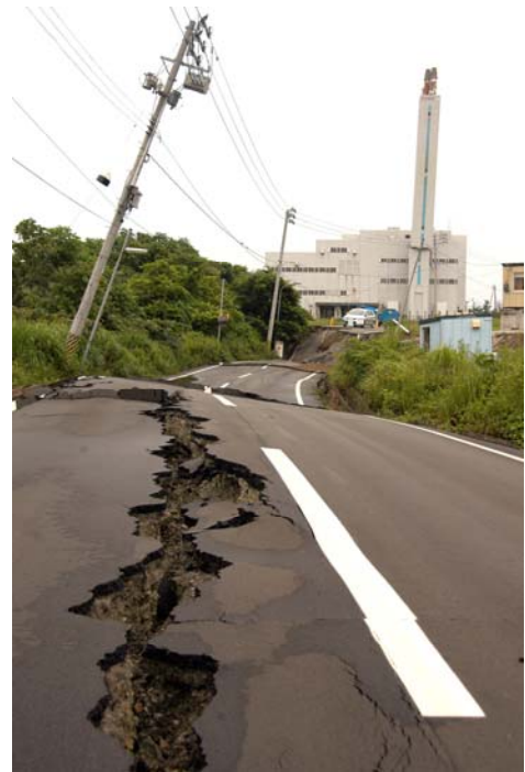
Figure 8: Failure of reinforced concrete stack and a large liquefaction-induced lateral spread on the north side of the Sabaishi River (Google Earth map site SP31, N 37.3939° E 138.5840°).
