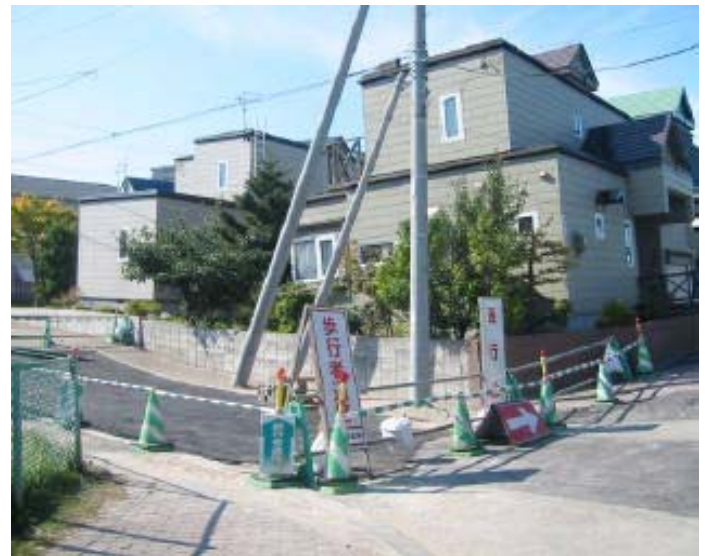
Figure 39: Damage to houses in Utsukushigaoka suburb of southern Sapporo from liquefaction induced settlement.
