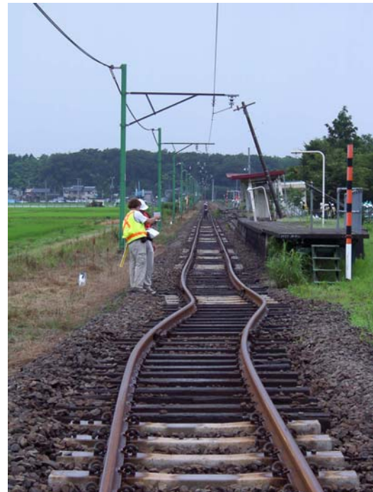
Figure 19: Lateral deformation of train tracks at Arahama Station (Site RK13; N37.40555° E138.60197°, 7/21/07)
