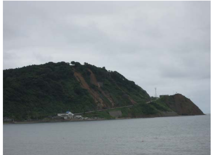
Figure 12: Coastal landslides on Highway 352 north of Kashiwazaki-Kariwa Nuclear Power Plant at road closure south of Route 373 (Google Earth map site RK34; N37.48455° E138.62435°; Photo taken 7/22/07).
