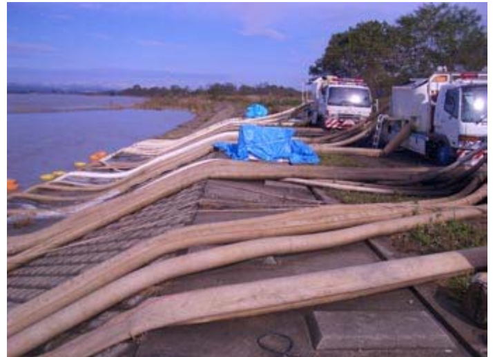
Figure 34: Emergency drafting of water from Shinano River for Nagaoka City Water Treatment Plant (photo: C. Scawthorn).
