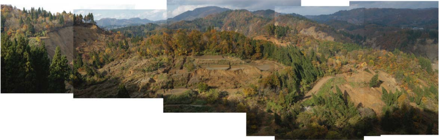
Figure 28: Deep rotational slump, indicated by a block of back-rotated trees and agricultural land, beneath an approximately 30m-50m foot high headscarp (photo mosaic: R. Kayen).
