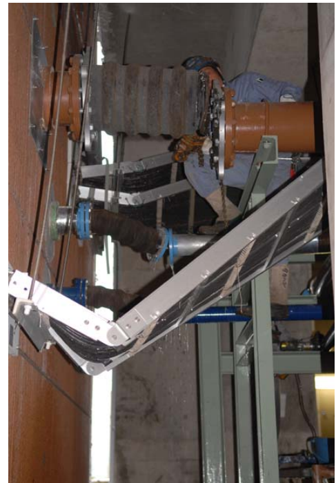
Fig. 6: Kashiwazaki Wastewater Treatment Plan on the south side of Sabaishi River near its outlet to the Sea of Japan (Google Earth map site RK9 RK9 N 37.38748 E 138.56587) Pipe breaks due to separation of two halves of building (Photo taken on 7/21/07).
