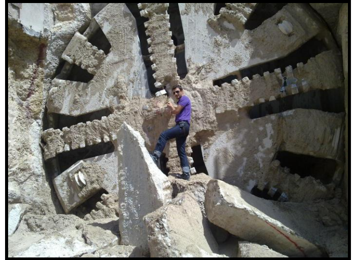
Fig. 15. Breakthrough of the machine of Esfahan Subway Project
