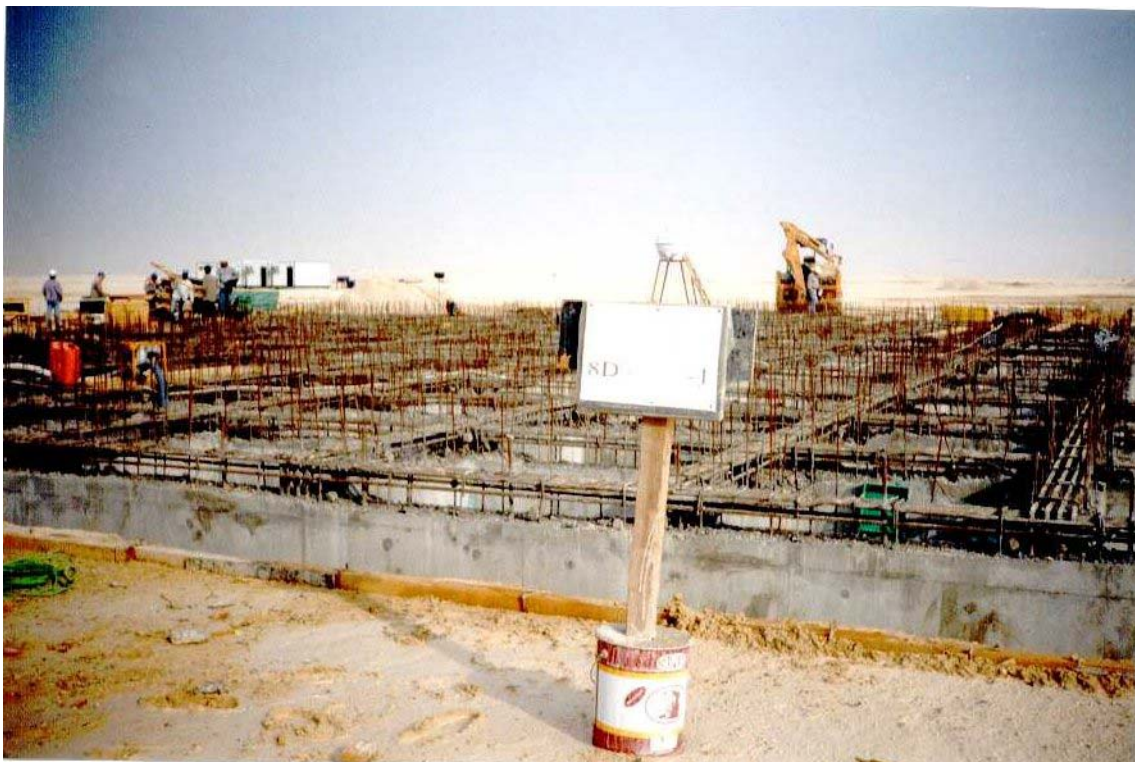
Plate: 2 Concrete placing in Stiffened Slab Waffle Foundation at the Site
