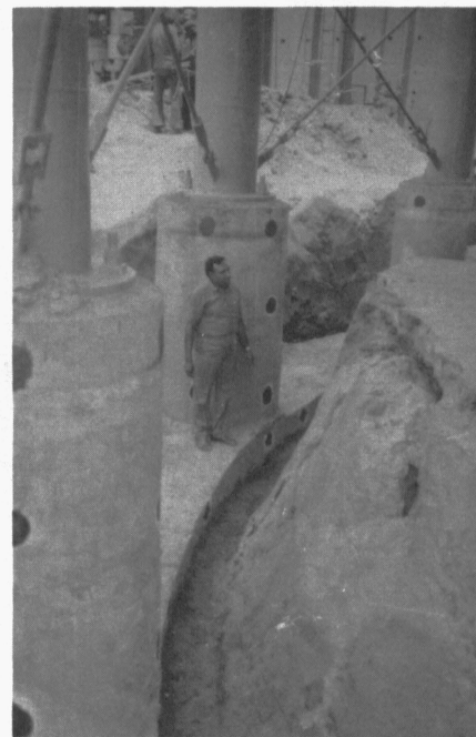
Fig. 2 - CONCRETE COLUMNS AND RING BEAM
