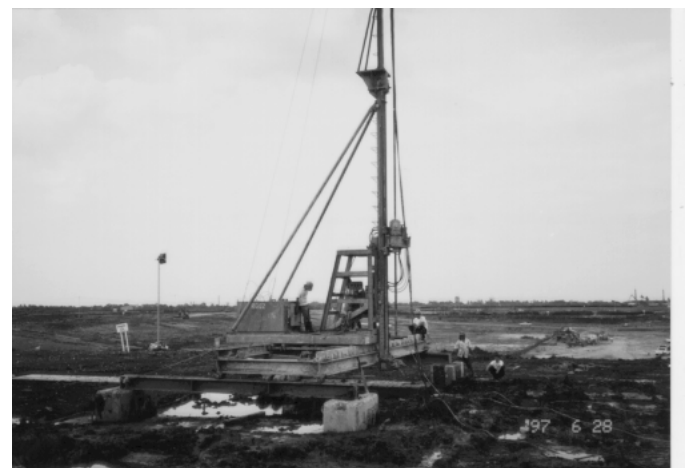
Fig. 5. Jet grouting method in construction site.
