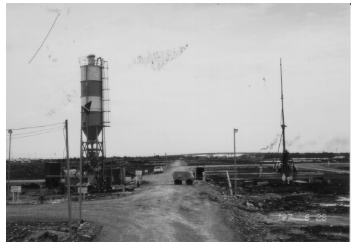
Fig. 4. Jet grouted installation at the site.
