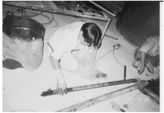
Fig. 8. Jet grouted coring.
