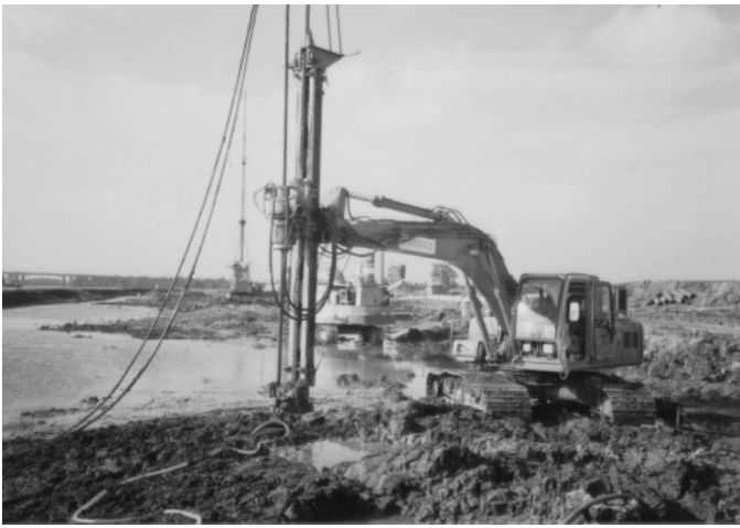
Fig. 6. Jet grouted machine during installation.
