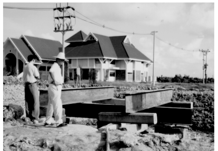
Fig. 10. Pile load test for inspection of jet grouted piles.
