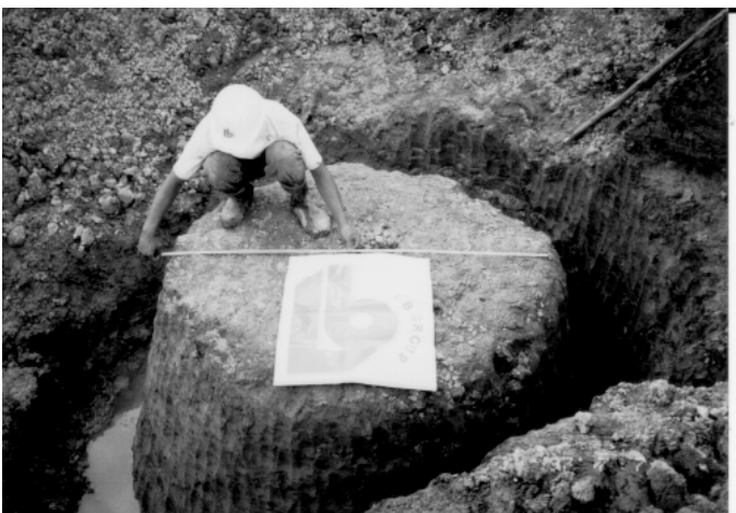
Fig. 7. Jet grouted piles after installation.
