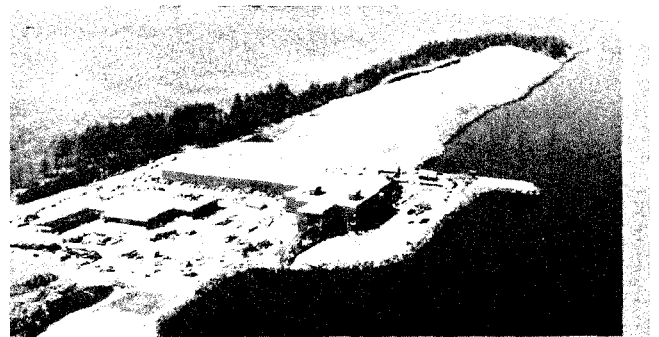
Fig. 1. Completed Mill, Looking North
