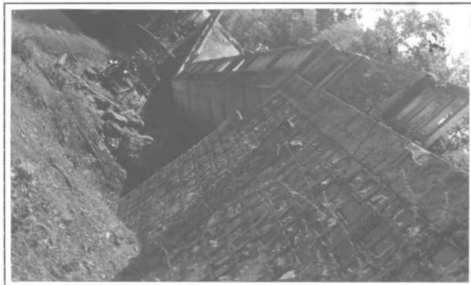
Photograph 2 Showing no damage signs in abutment and wings
