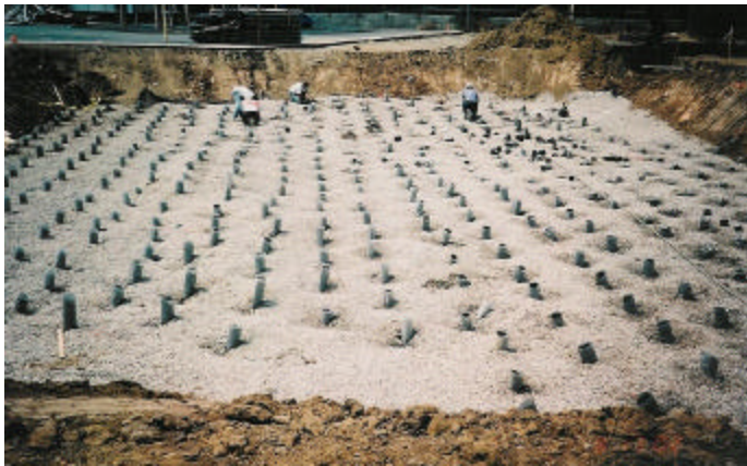
Fig.6. Trimming drains to uniform height at Barnard Elementary School Library.
