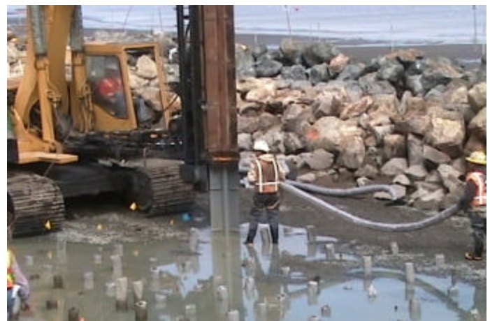
Fig. 3. Installing Earthquake Drains at Bay Bridge.
