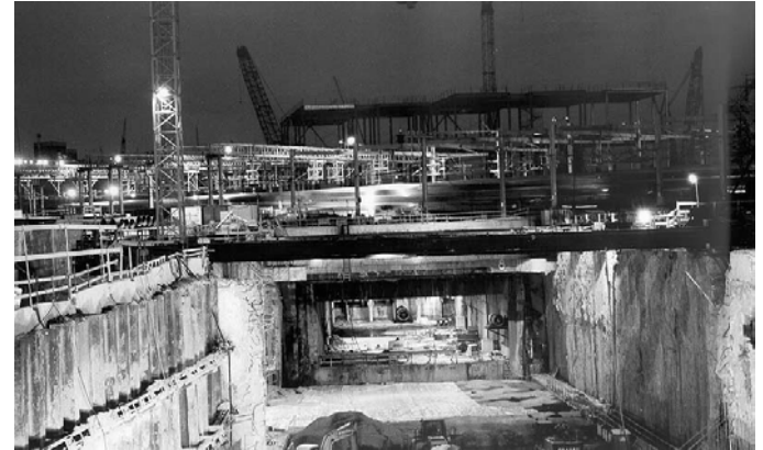
Fig. 11. Completed West Bound Tunnel Jacking Pit
