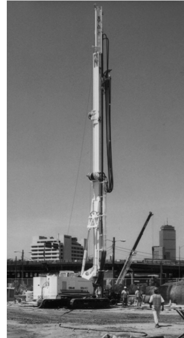
Fig. 7. Soilmec CM-40J Drill Rig performing Jet Grouting
