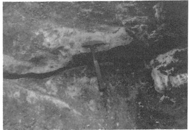
Fig. 4. Characteristic joint in marly limestone
