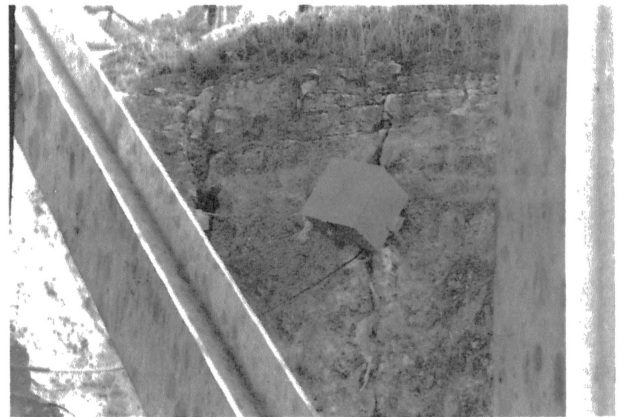
Fig. 5. Installation of a crack displacement transducer on joint walls
