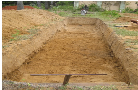
Fig: 2 Excavated Pavement Stretch
