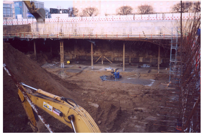
Fig. 6. General overview of excavation at “-3” level stage.
