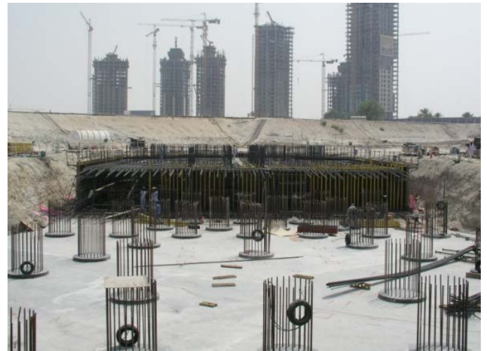
Fig. 5: Individual Wing of Tower Raft
