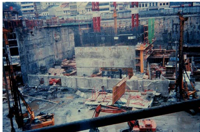
Fig. 18: Plaza Rakyat Office Tower Below-Grade Construction
