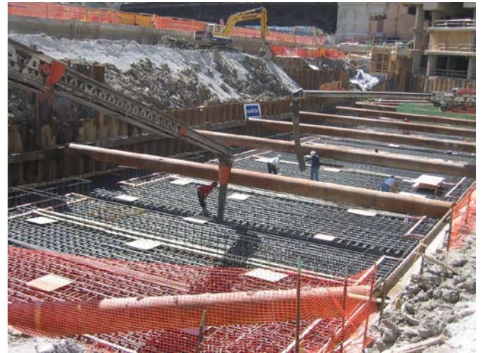
Fig. 12: Mat Foundation Construction
