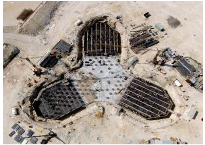
Fig. 4: Tower Raft Under Construction
