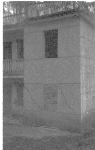
Fig 4. Crack Failure of Lower Houses on The ECRC
