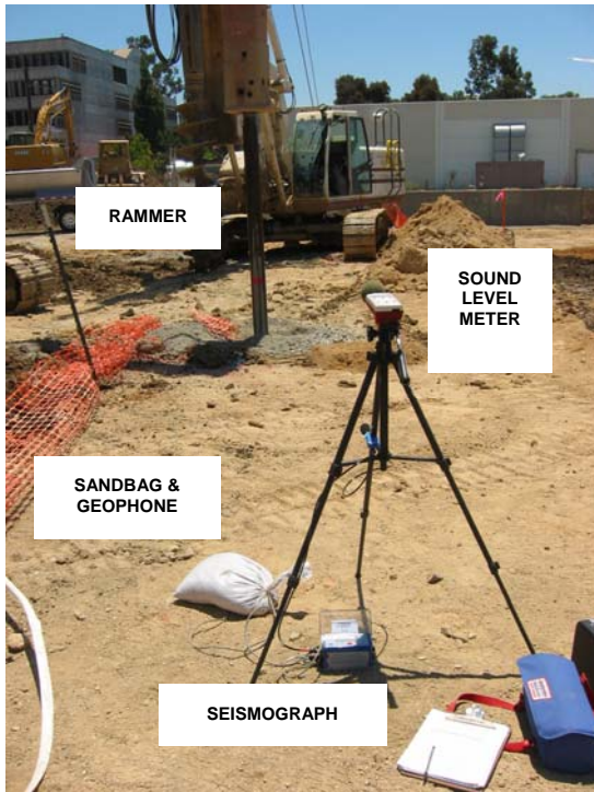
Fig. 4 Photograph showing typical instrumentation set-up.
