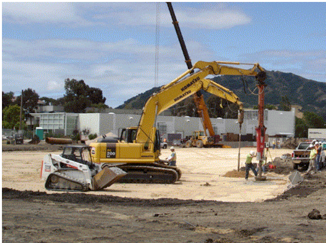
Fig. 2. Typical RAP installation equipment.
