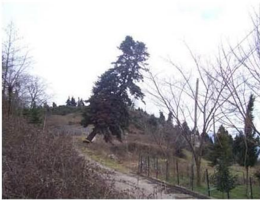
Fig. 5. Kerasia slide. Photos at 28/12/2010. (a)-(b) Top of the slide, (c) oblique tree illustrating slide movement.
