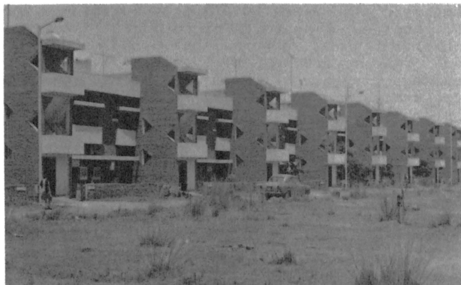
Fig. 3. View of Completed Accommodations
