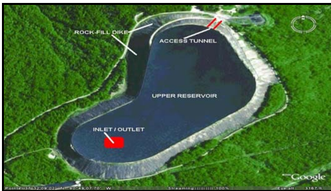
Figure 4. Aerial view of Upper Reservoir.
