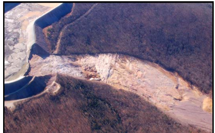
Fig. 1. The upper reservoir breach and a portion of the flow path (photo courtesy of J. Spooner, 2005)
