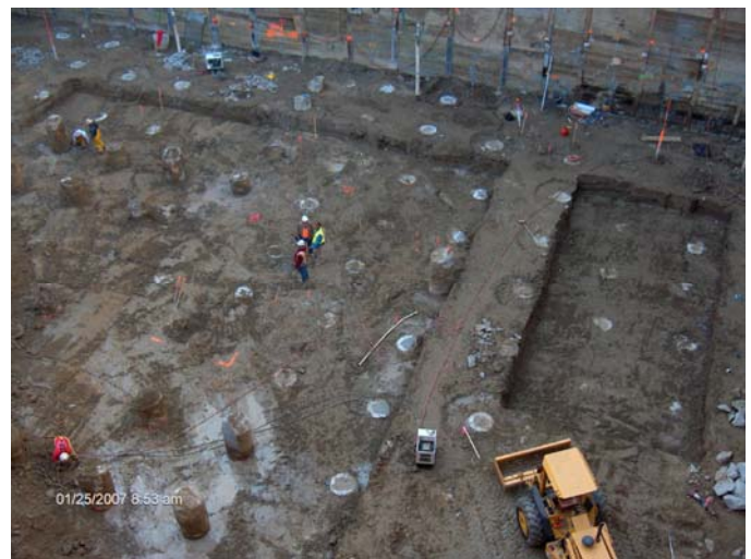
Fig. 8. Trimmed LCCs and reinforced foundation subgrade
