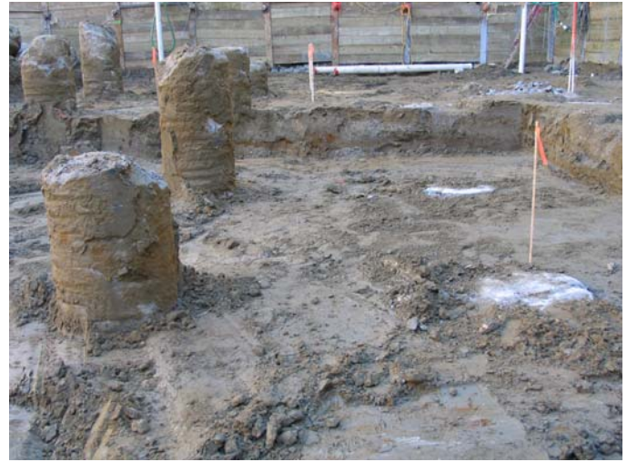
Fig. 7. Tops of LCCs before and after trimming
