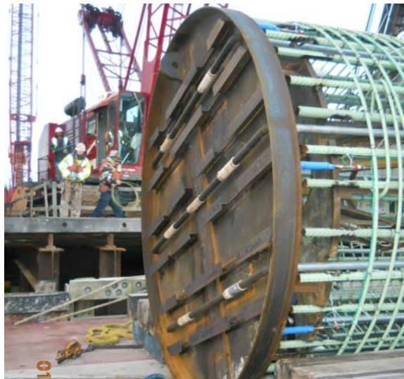
Fig. 11. Tip grouting apparatus installed at the cage tip.
