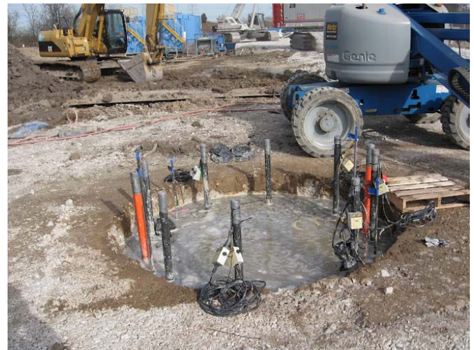
Fig. 8. Installed Test Shaft CTS-1
