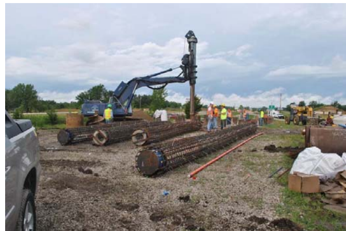
Fig. 9. Multiple O-cell load test assemblies ready for installation.
