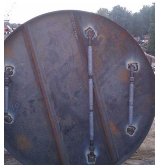
Fig. 2. Malcolm Drilling's tube-a-manchette system
