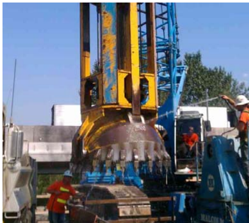
Fig. 3. Malcolm Drilling's clam shell grab
