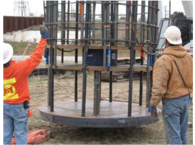
Fig. 7. O-cell and tube-a-manchette system in rebar cage
