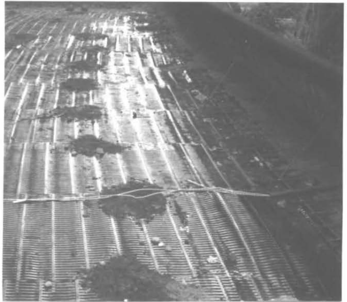
Photo 3: Geosynthetic reinforcement and framework Thermolectric cells
