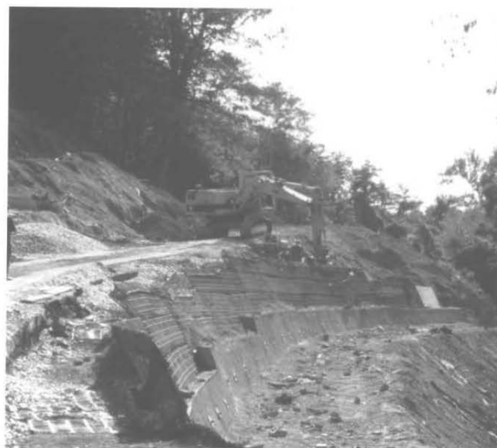
Photo 1: General view of the structure
