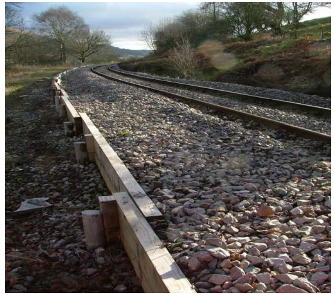
Fig. 9 View of finished Grundomat piles
