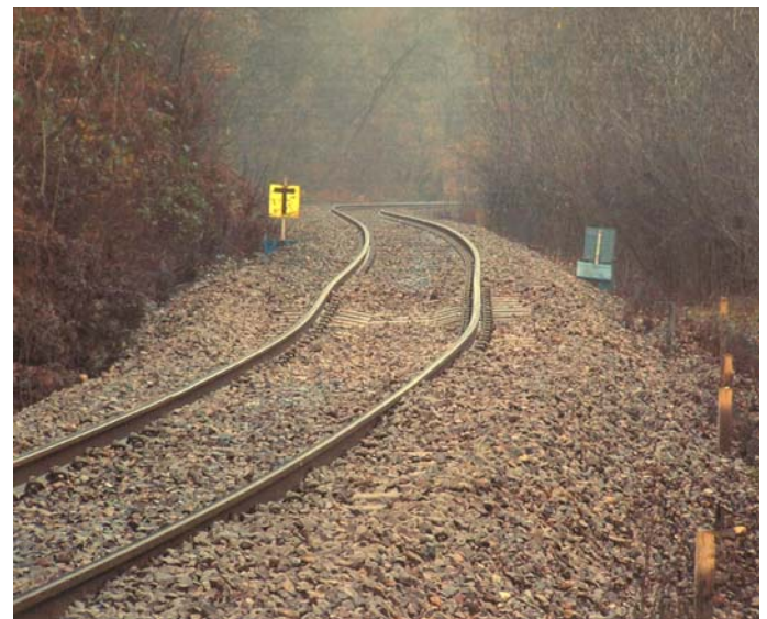
Fig. 3 View of track looking north, November 2004
