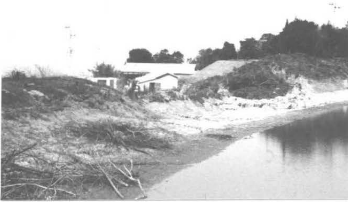
Photo. 1 Liquefied earth dams of Grade 4 (Ichinomiya-cho in Awaji Island)
