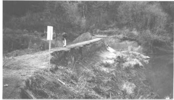
Photo. 2 Slid earth dams of Grade 4 (Ono City in Honshu Island)
