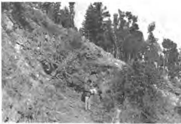
Fig.2 Tilting of Trees on Slope
