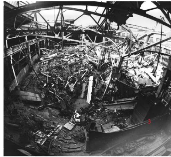
Fig. 3. Sinkhole in Dzerzhinsk, Russia, 1991.
