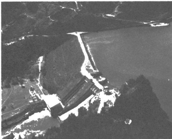
Figure 4. Matahina Dam (D.L. Homer DSIR)
