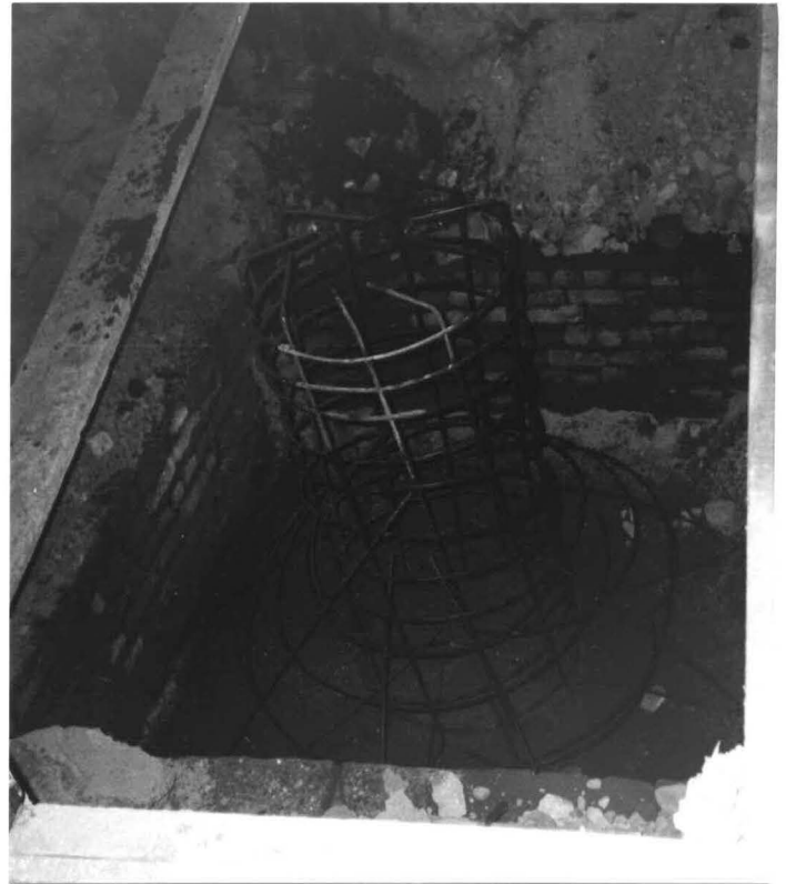
Fig. 2 End bearing pile reinforcement
