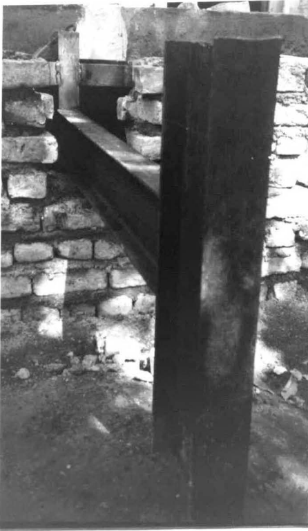
Fig. 6 Connection between stiffener and column
