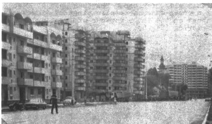
Fig.1 Uneven settlements of the block of flats
