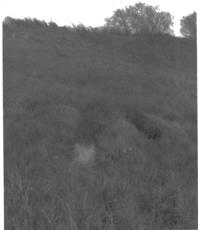
Fig. 1 Seepage at the innerslope
