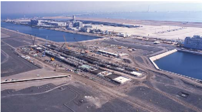
Fig. 27. Underpass under construction
