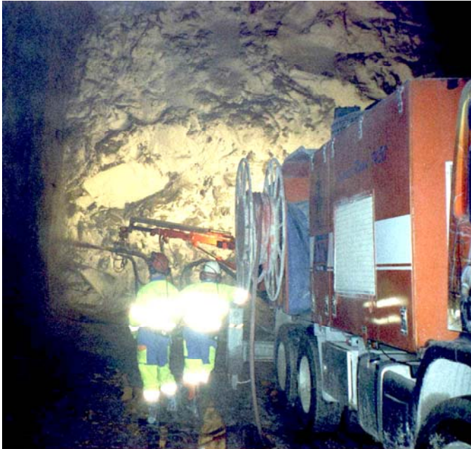
Fig 9. Shotcreting of the blasted tunnel end in October 2002.
