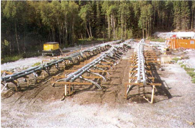
Fig. 7. Freezing installation on the ground surface, summer 2002.
