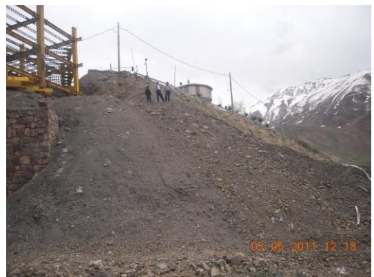
Fig.21. Loose dumped materials
