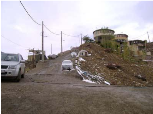
Fig. 3. Existing access road
