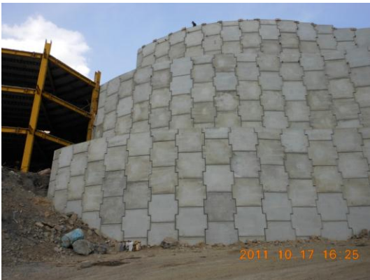
Fig. 23. Three steps walls
