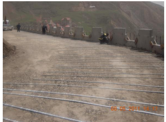
Fig.16. Connecting galvanized strips to concrete panels
