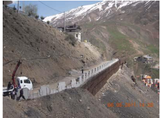
Fig.15. Concrete panel installation
