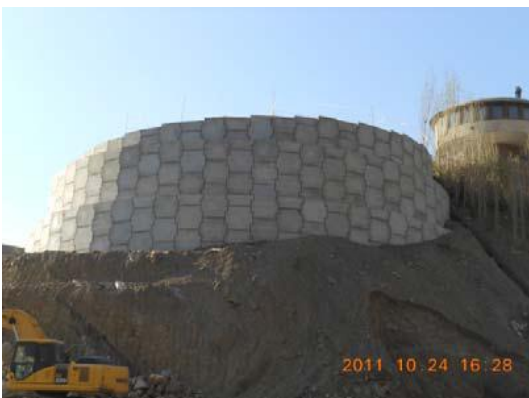
Fig.24. Reinforced earth walls in the curve
