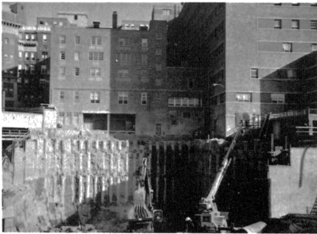
Figure 7. Hospital Area During Construction
