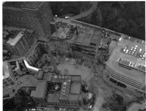
Figure 1. Aerial View of Project During Early Construction Phase
