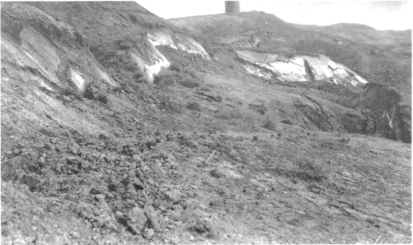
Figure 7 - Slickensided Scarp of Slide 4, 2 Oct 1934 (Photo 34/1184)
