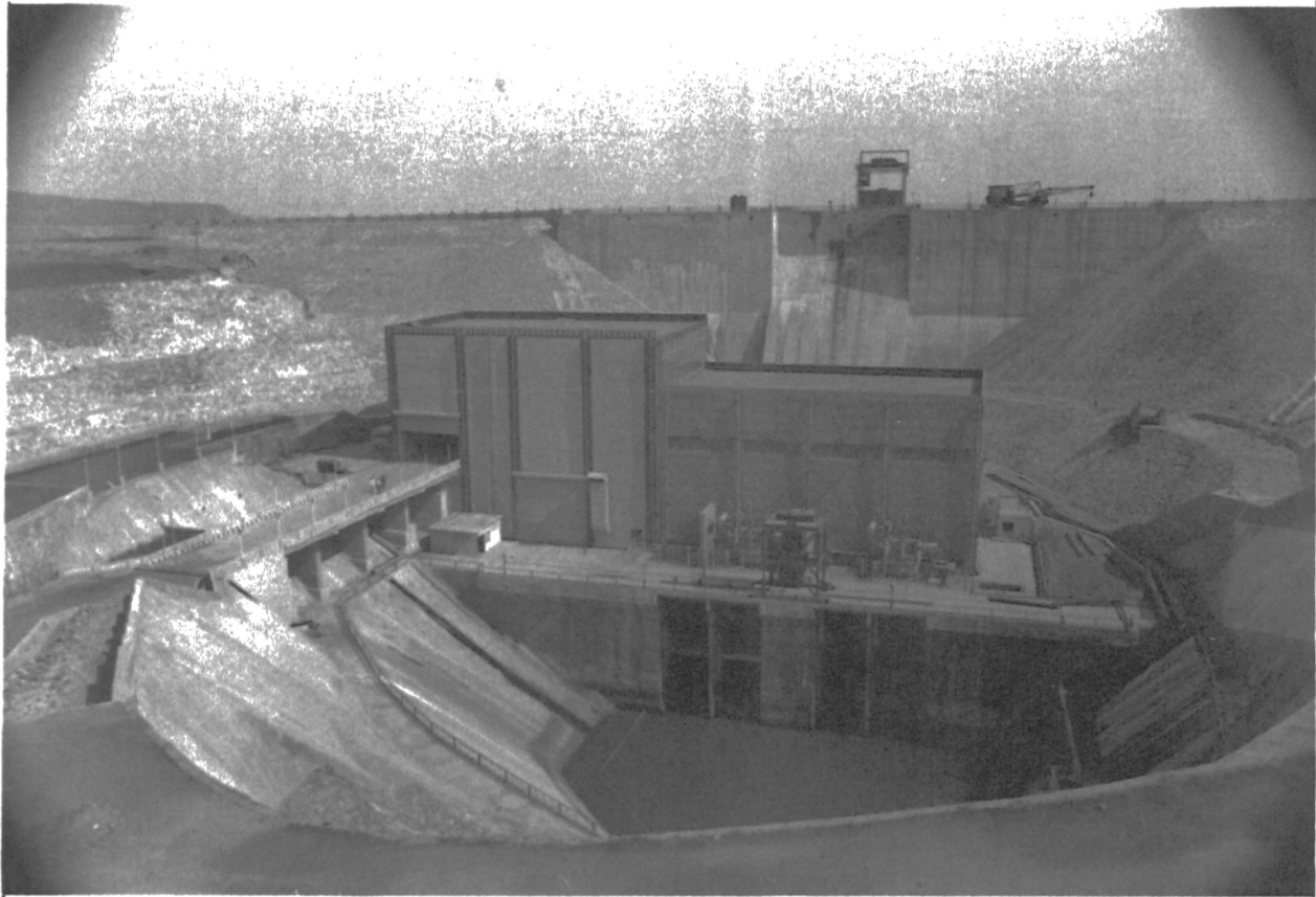
Fig. 7 General view of Power House.
