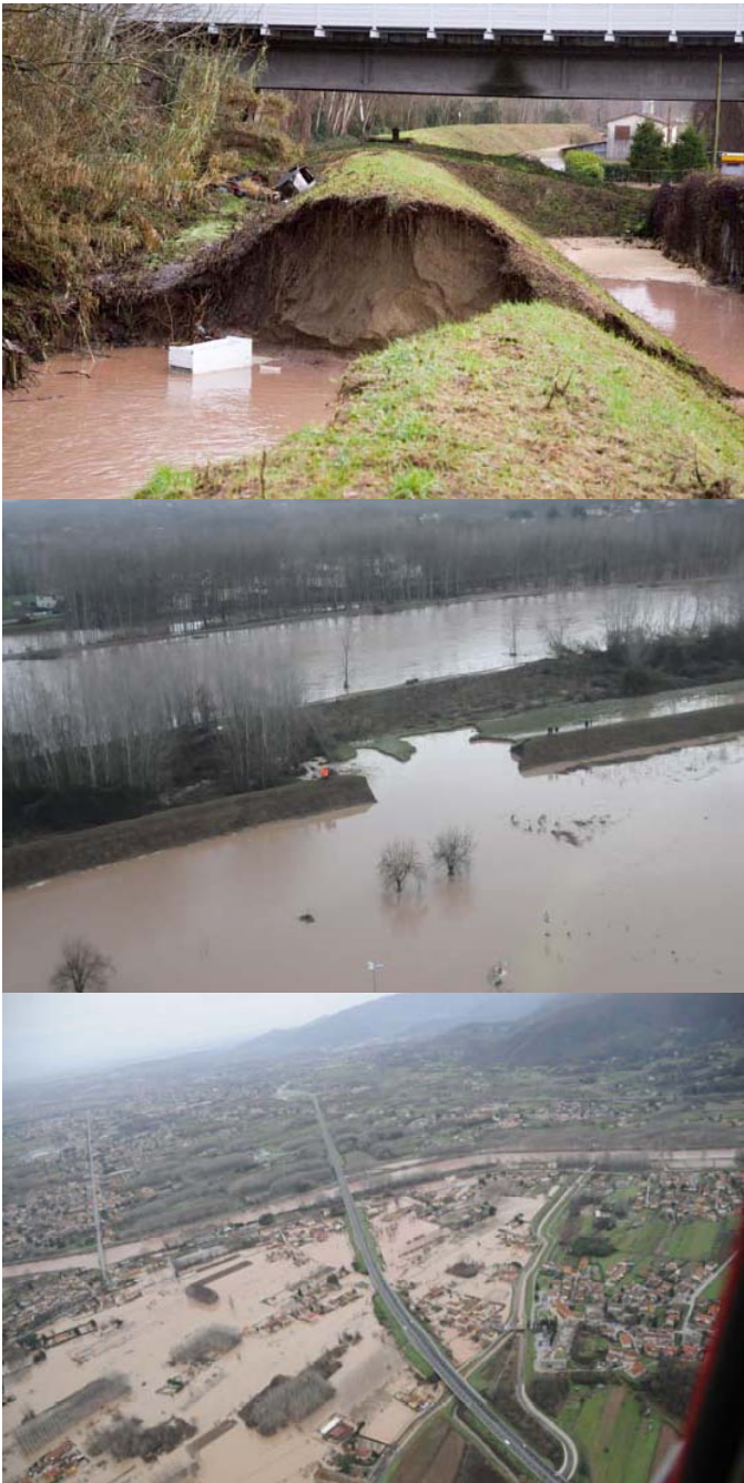
Fig. 3. Failures and flooded areas in the District of Lucca (Pictures: Italian Civil Service).
