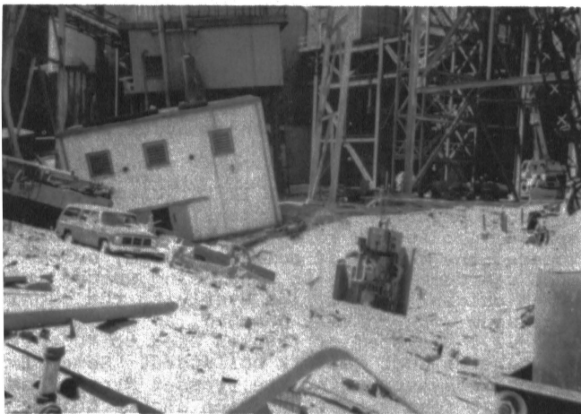
Fig. 2 Surface Deformation Resulting from Pipeline Collapse
