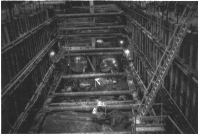
Fig. 8 Excavation and Installation of Retaining System
