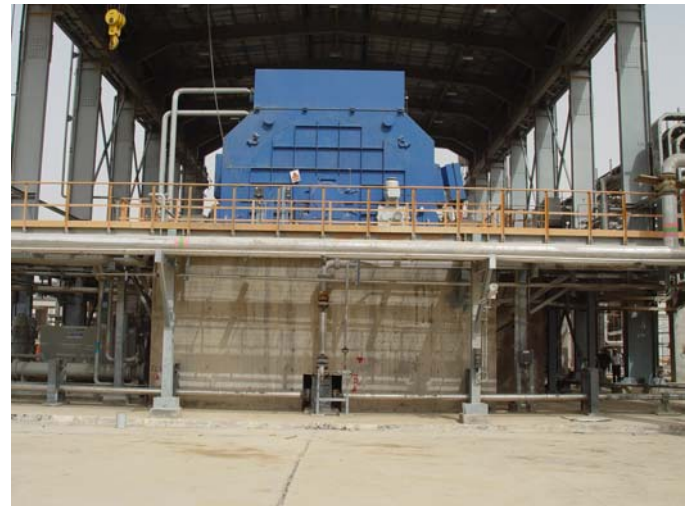
Figure.1. The view of the compressor's concrete foundation
