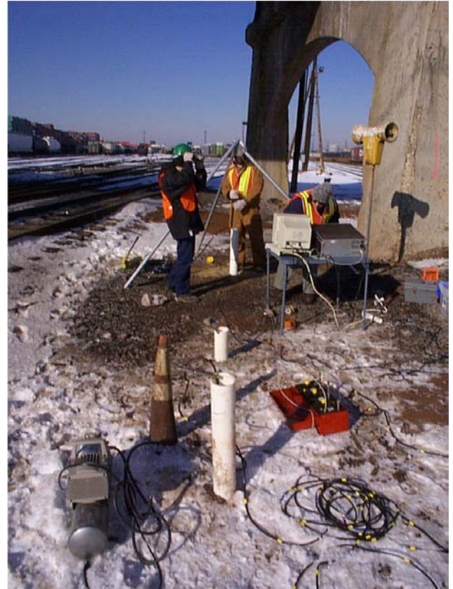
Fig. 5. Crosshole Test at Doremus Avenue Bridge
