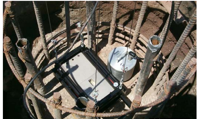
Fig. 15. Drilled Shaft Test at Doremus Avenu Bridge
