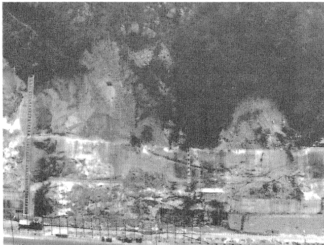
Figure 2 Oblique aerial photograph after failure (June 1982)
