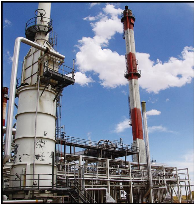
Fig. 1. Steel stack view
