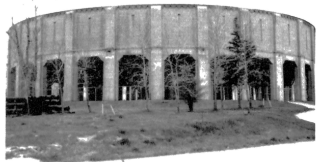
Fig. 1. Taylor Park Water Reservoir
