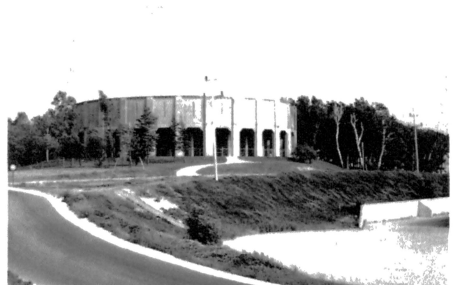
Fig. 2. Existing Taylor Boulevard Cut
