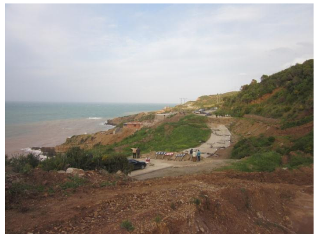
Fig.9. Overview of landslide Assoumeth RN24 PK 226+ 300
