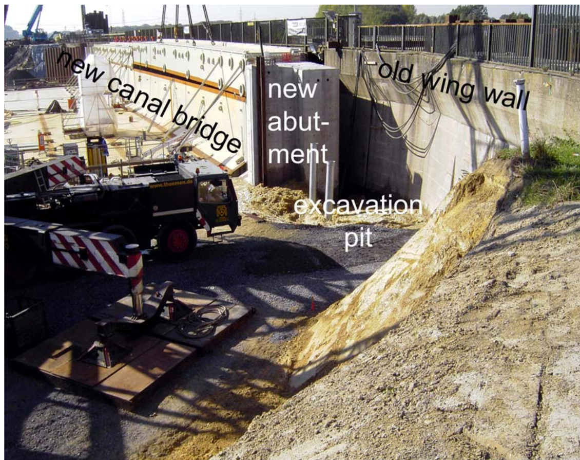
Fig. 4: View of the construction pit between the two abutments
