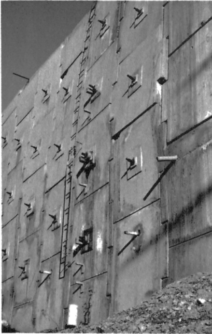
Fig. 3 Nailing facing
